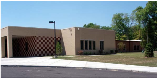
Westbrooke Village Elementary School
